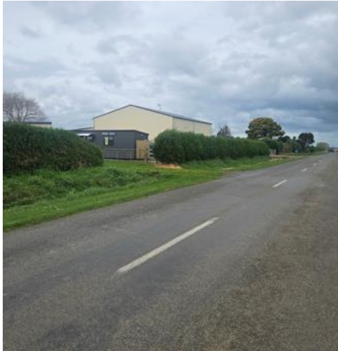
Figure 3: View from road boundary looking south east (Applicant photograph 29/08/24).
