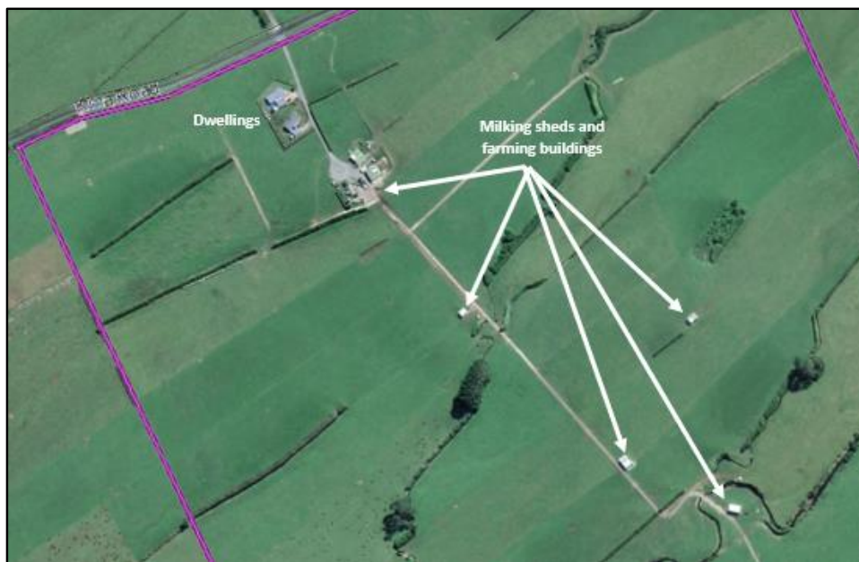
Figure 1: Existing buildings and associated accessways (Source: Google Earth).
