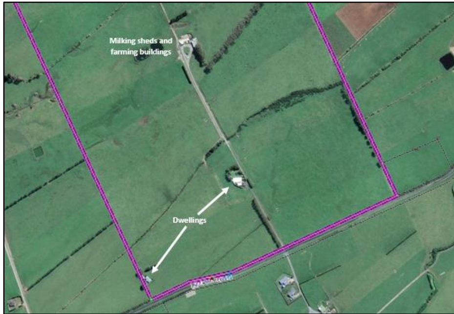
Figure 2: Existing buildings and associated accessways (Source: Google Earth).
