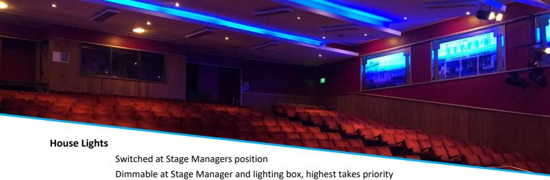
RGB LED lights installed in the ceiling steps and wall art are switched in the lighting box. These are normally DMX controlled through the lighting desk or can be set on a slow colour scroll by request to the Venue Tech.
