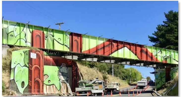
Northbound view of the Hawera rail bridge
